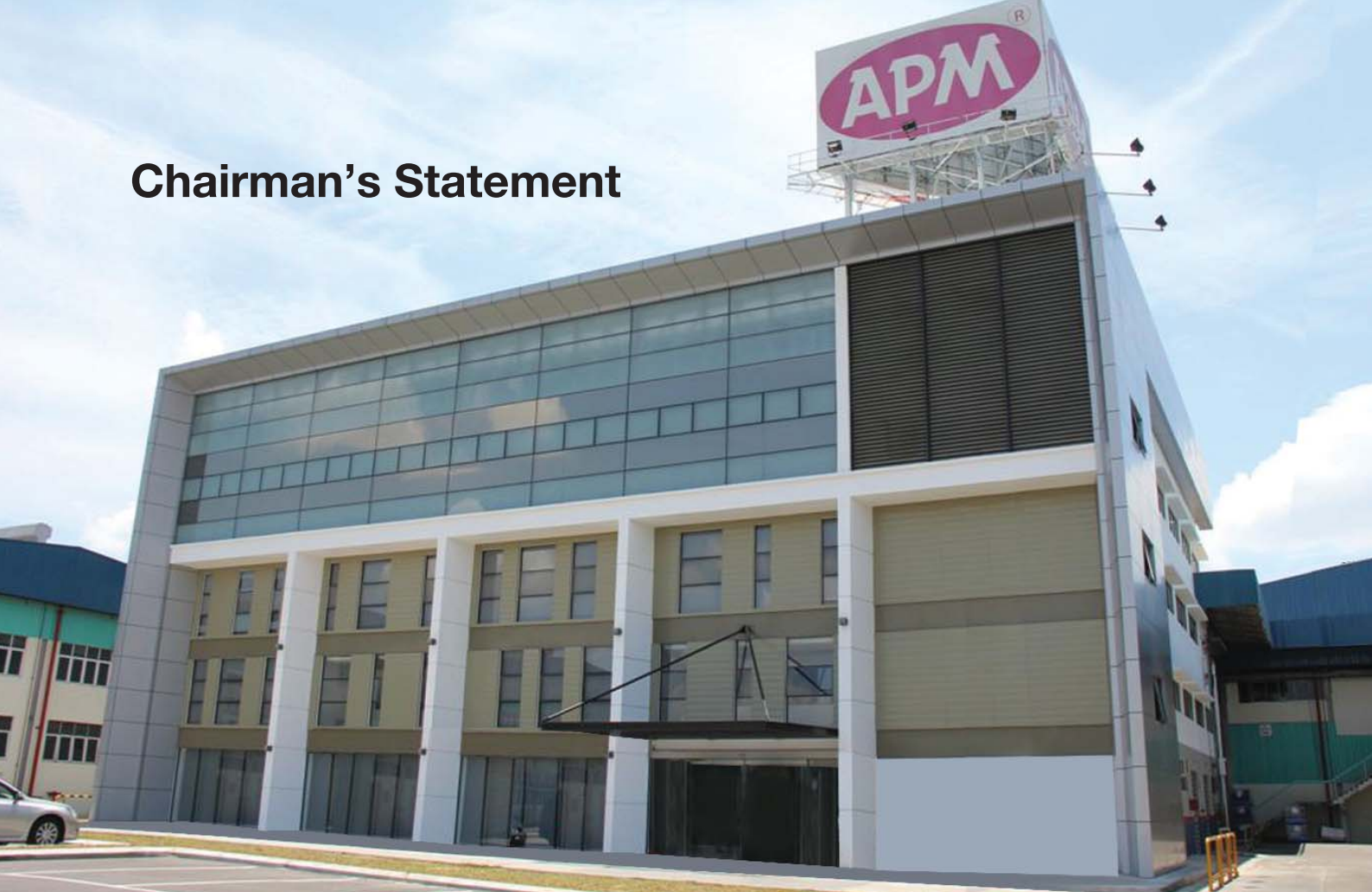
New Corporate Head Office, Port Klang
