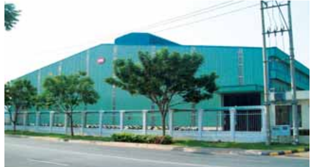
Newly constructed plant in Vietnam
